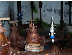
Detecting leakages in pipes by high tech instruments allowing rapid and accurate intervention of maintenance teams.
